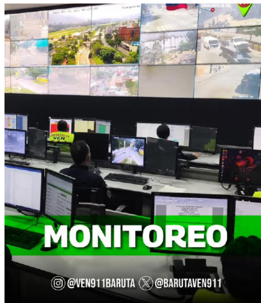
Monitoring room at the VEN911 Baruta headquarters. (Source: Ven911baruta on Instagram 37 )
